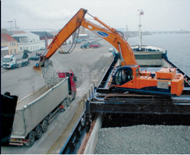
DISCHARGING SPLIT TO LORRIES
