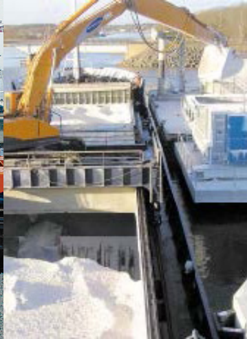
DISCHARGING TO HOPPER
