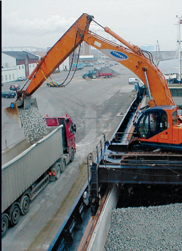
DISCHARGING SPLIT TO LORRIES
