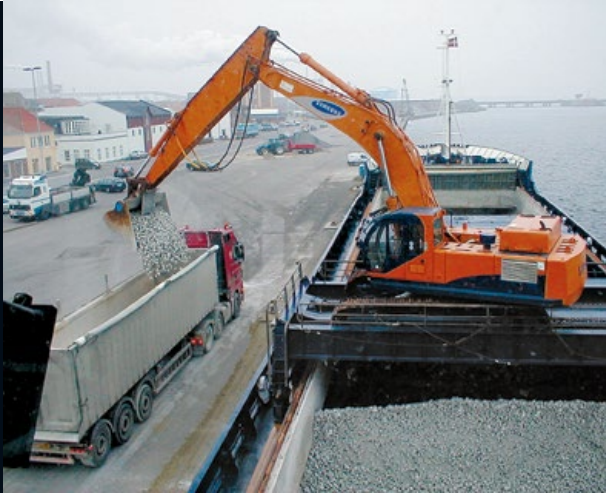
DISCHARGING SPLIT TO LORRIES
