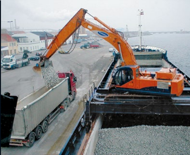
DISCHARGING SPLIT TO LORRIES
